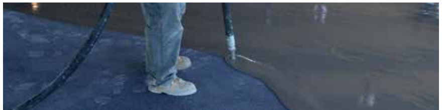
ARDEX HC 100™ High-Capacity Self-Leveling Underlayment ARDEX HC 100R™ High-Capacity Rapid Self-Leveling Underlayment
